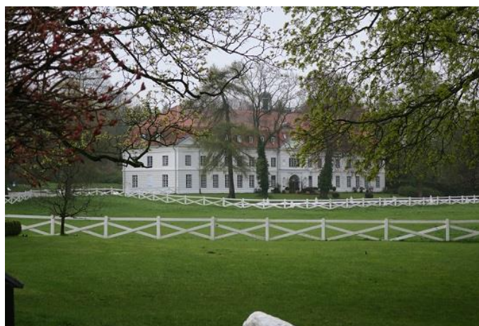
Figure 8: One of Panker Estate's many houses (Germany)
