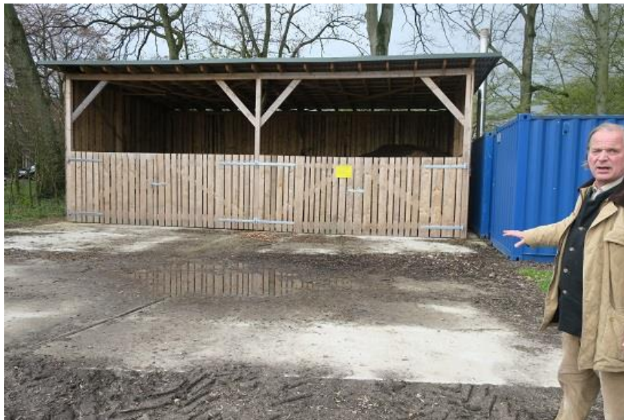
Figure 32: Enno Freiherr Von Ruffin’s woodchip bunker for his subsidy-driven heating system. I was most impressed by the bunker’s simplicity and low installation cost (Germany)
