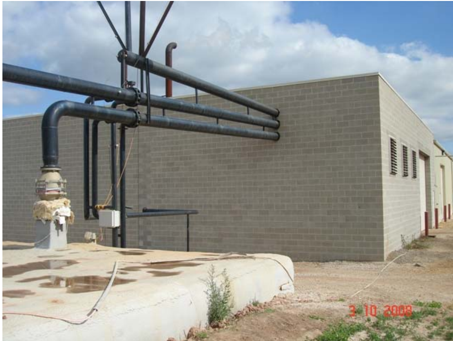
Image 19: the CHP plant at Holsum Elm Dairy
