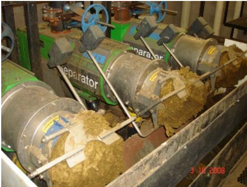
Image 20: Separation of solids from digestate stream
