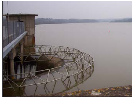
Weir Wood Reservoir at capacity
